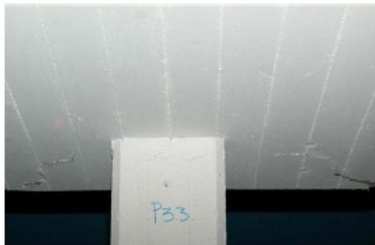
Figure 24. Floor 3 (below): slab crack detail around the perimeter of column P3
